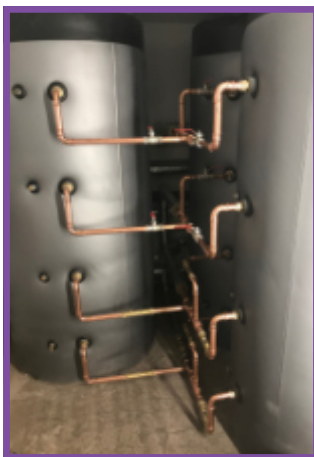
Photos: New pipework and hot water storage in the new plant room below the Bill McDonald Upper Hall
